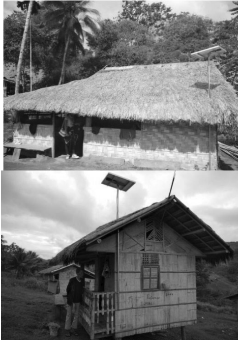
Diagram 8: Roof-through Pole mounted installations on thatched roof
