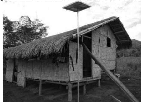
Sample Roof-side Pole mounted installation
