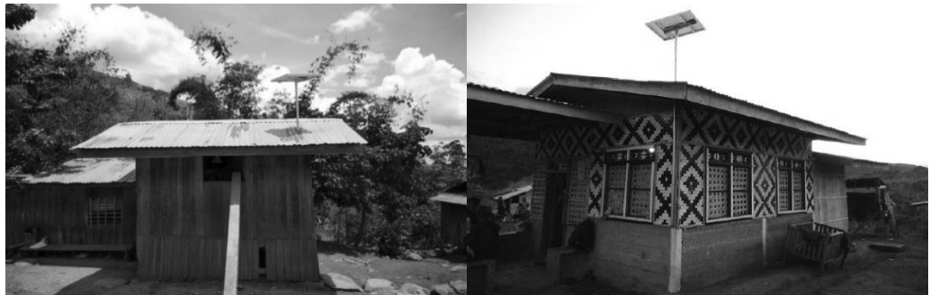
Diagram 7: Roof-through Pole mounted installations on GI roofs
